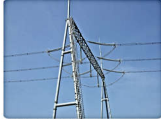
管型变电站架构 35kV-1000kV Tubular Steel Structure in Substation 35kV-1000kV
