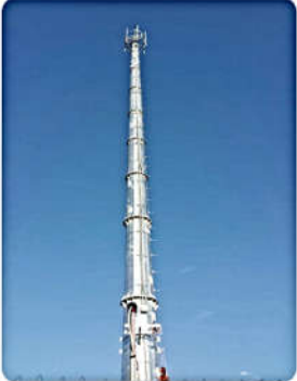
单管信号塔 Tubular Telecommunication Tower
