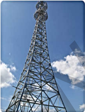
电信/通讯塔 Lattice Telecommunication Tower
